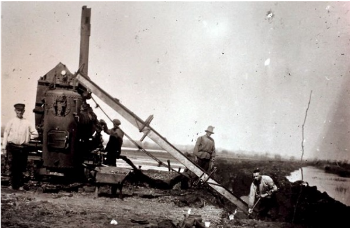
Machinale turfwinning in de Oostpolder
